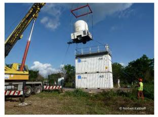
The X-band radar was positioned on top of two containers allowing to do horizontal scans and detection of precipitation in a radius of about 100 km.
